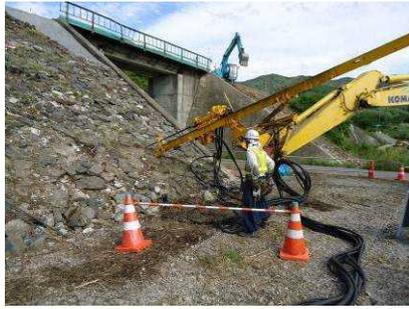
(a) Insertion of the rod into the embankment
