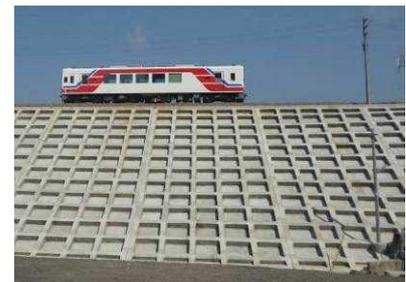
(b) Inland side slope covered with a cast in place concrete lattice frame
