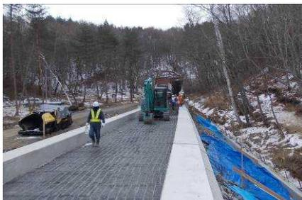
Photo 7 Side slopes of the embankment and the geogrid layer.
