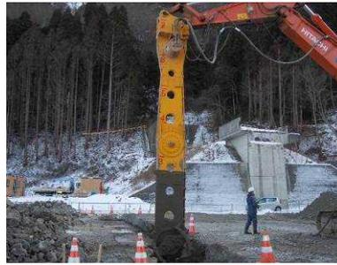
(b) Construction of measures to prevent scour by overflowing tsunami
