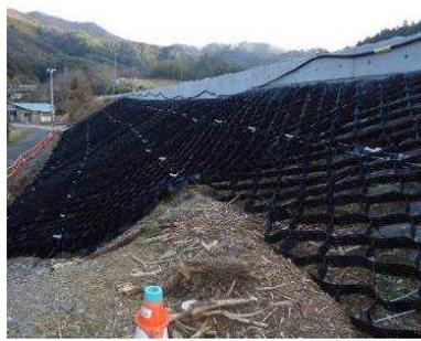
(b) Arrangement of geocell on the slope
