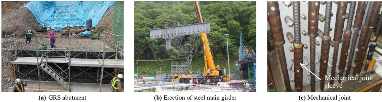
**Photo 5** Construction of Haipe-sawa GRS integral bridge.
