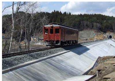
(a) Seaside slope covered with a cast in place concrete facing
